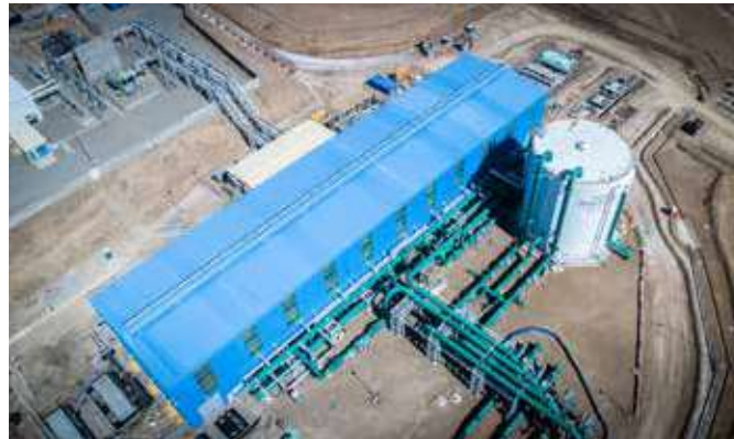
Escondida Water Supply Expansion (EWSE), Chile.
